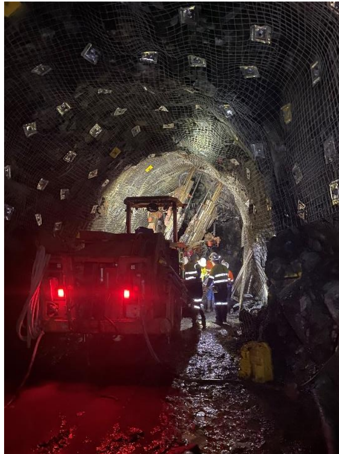
Ground support installation in the Otter decline
